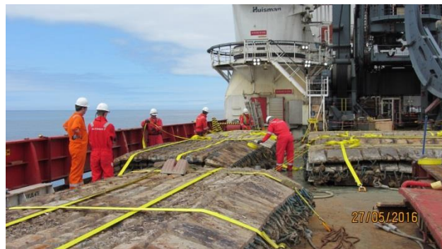
Figure 9.3.1: Mattresses Recovered and Secured on-deck
