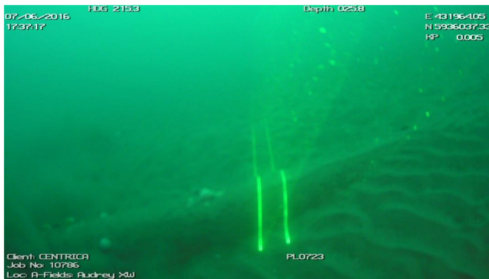
Figure 4-10: Exposed pipeline between KP0.113
